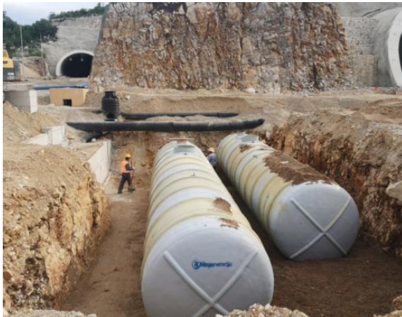
(c) Installation of Oil-Water Separators
