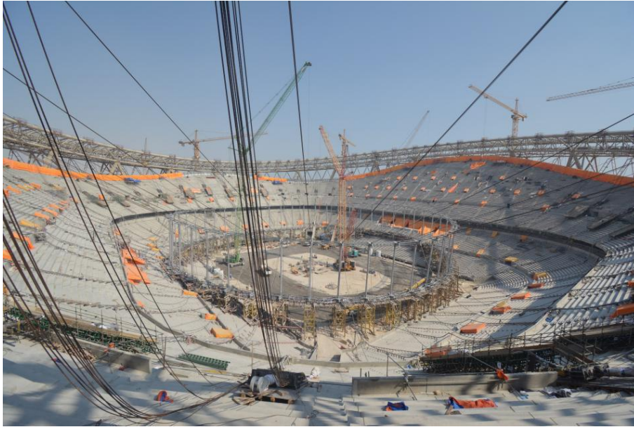
Figure 7- 2. The Construction of the Cable Net Roof
