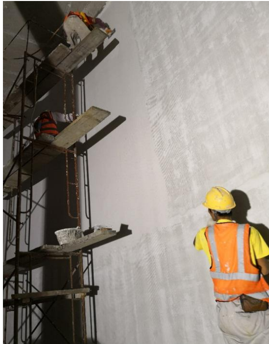
Figure 3- 3. Application of Sika, Waterproofing Coating
