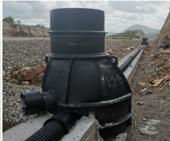
(b) Connection Between the Inspection Well and Drainage Pipes
