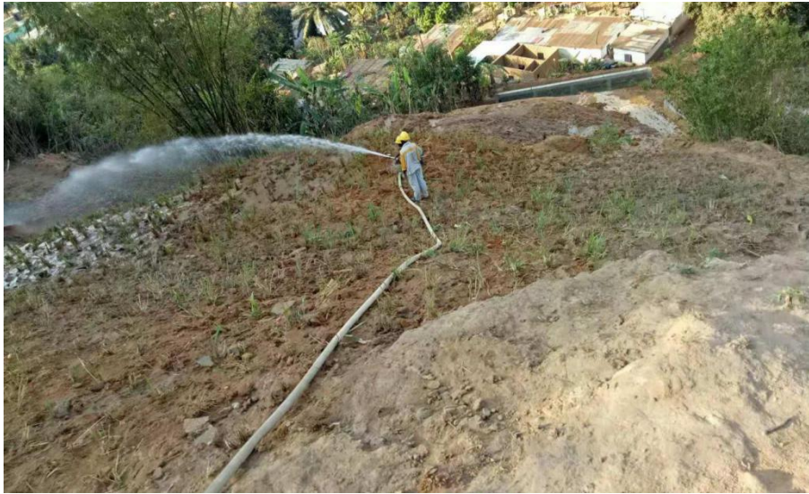
Figure 3- 4. Use of Waste Bituminous Concrete to Protect Steep Road Segments from Runoff
