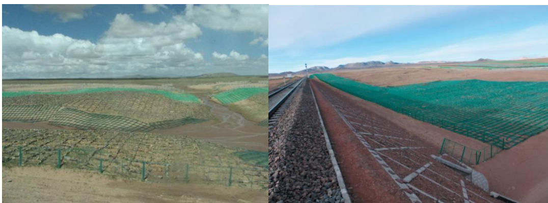
Fig. 4.15 Sand-fixing grids along the Qinghai-Tibet Railway
