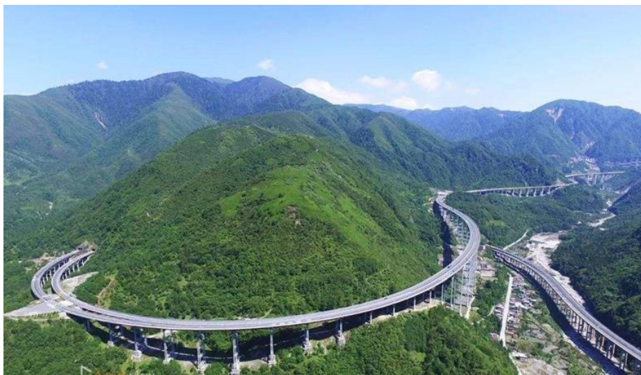
Fig. 4.14 Highway in the section with spiral route development
