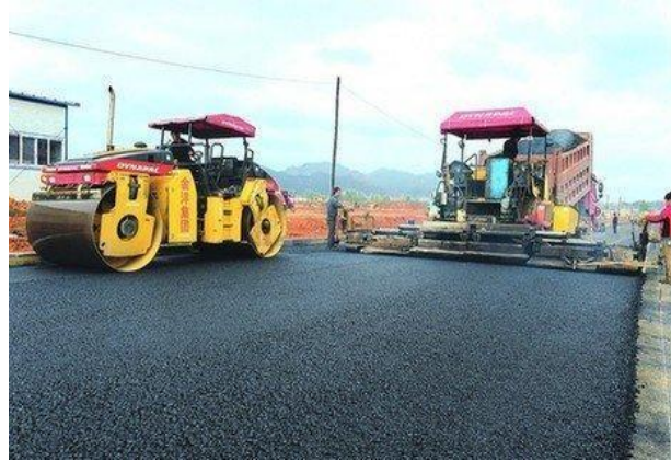
Fig. 4.30 The warm mixing technology of asphalt mixture in the Hainan Wanning-Yangpu Expressway Project has significant energy-saving effects
