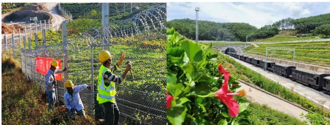
Fig. 4.18 Elephant protection fences along and picture of Yuxi-Mohan Railway
