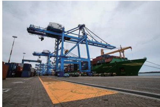
Fig. 62 No. 19 berth of Mombasa Port
