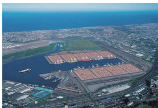
Fig. 61 Aerial view of Mombasa port
