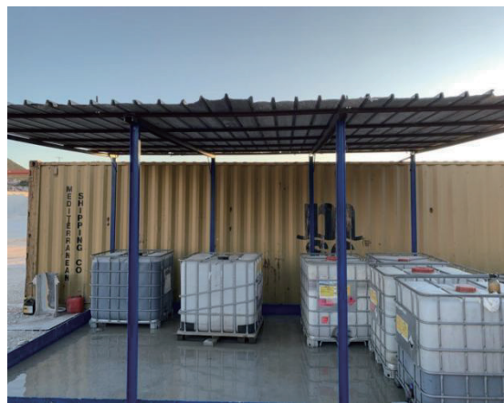
Fig. 44 Classified collection and storage of hazardous wastes
