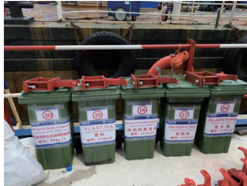
Fig. 43 Classified collection of construction waste in the construction area
