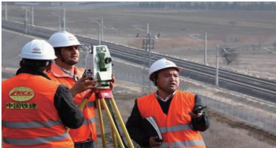
Fig. 4 Tunnel Construction Survey of Ankara-Istanbul High-Speed Railway
