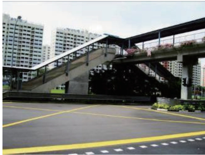
Figure 83 pedestrian overpass outside the bus terminal
