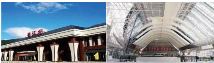
Fig. 9 Pu 'er Station and Xishuangbanna Station
