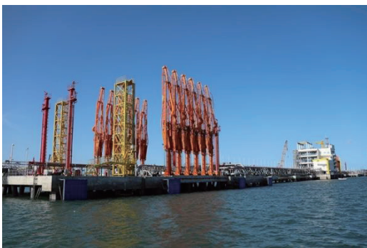
Fig. 63 Oil terminal of Mombasa Port
