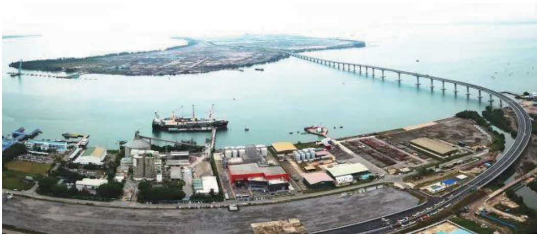
Fig. 27 PMB Bridge in Brunei
