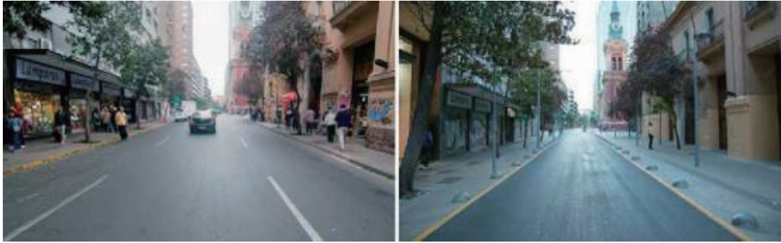
Fig.92 Downtown Santiago, a street was changed from three lanes to single lane, widening the sidewalks on both sides.
