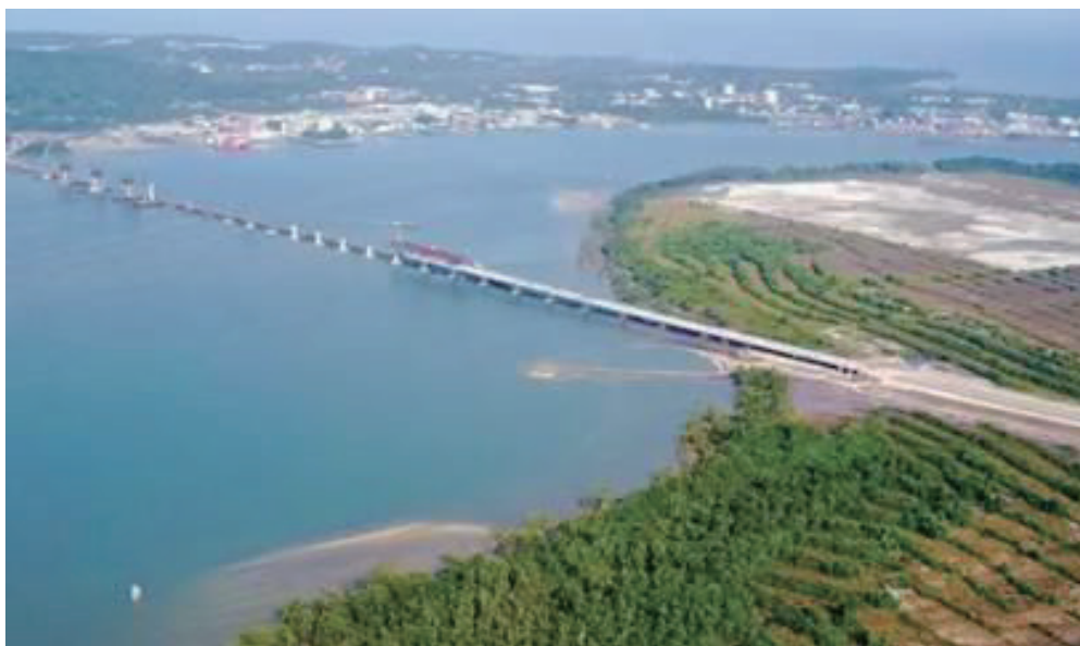
Fig. 30 Brunei PMB sea crossing bridge
