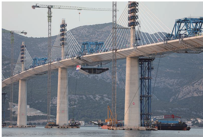
Fig. 33 Closure of Pelješac Bridge
