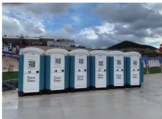
Fig. 47 recyclable mobile toilets are set at the construction site
