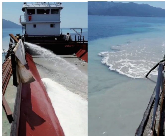
Fig. 35 Discharge of drilling slag by ships in designated sea area
