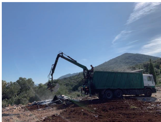
Fig. 46 Classified storage and centralized treatment of construction waste by professional companies
