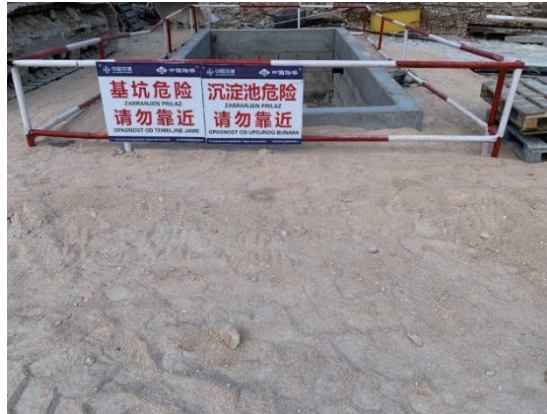
Fig. 41 Sedimentation tank for four stage sewage
