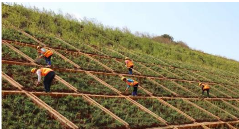
Figure 10.5 Greening works for China-Laos Railway
