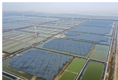
Fishery-solar Hybrid Projects for PV Power Generation in Nantong City, Jiangsu Province 72
